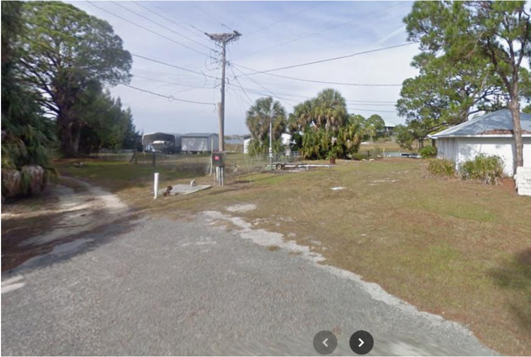
LS 16 - Corner of SW 120 th Place and SW 165 th Terrace
